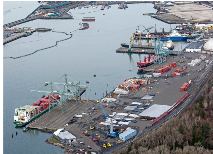
Conceptual image showing the cargo transit shed relocated to the east near the rail tracks and a strengthened South Terminal able to accommodate two, 100-foot gauge ship to shore cranes.
