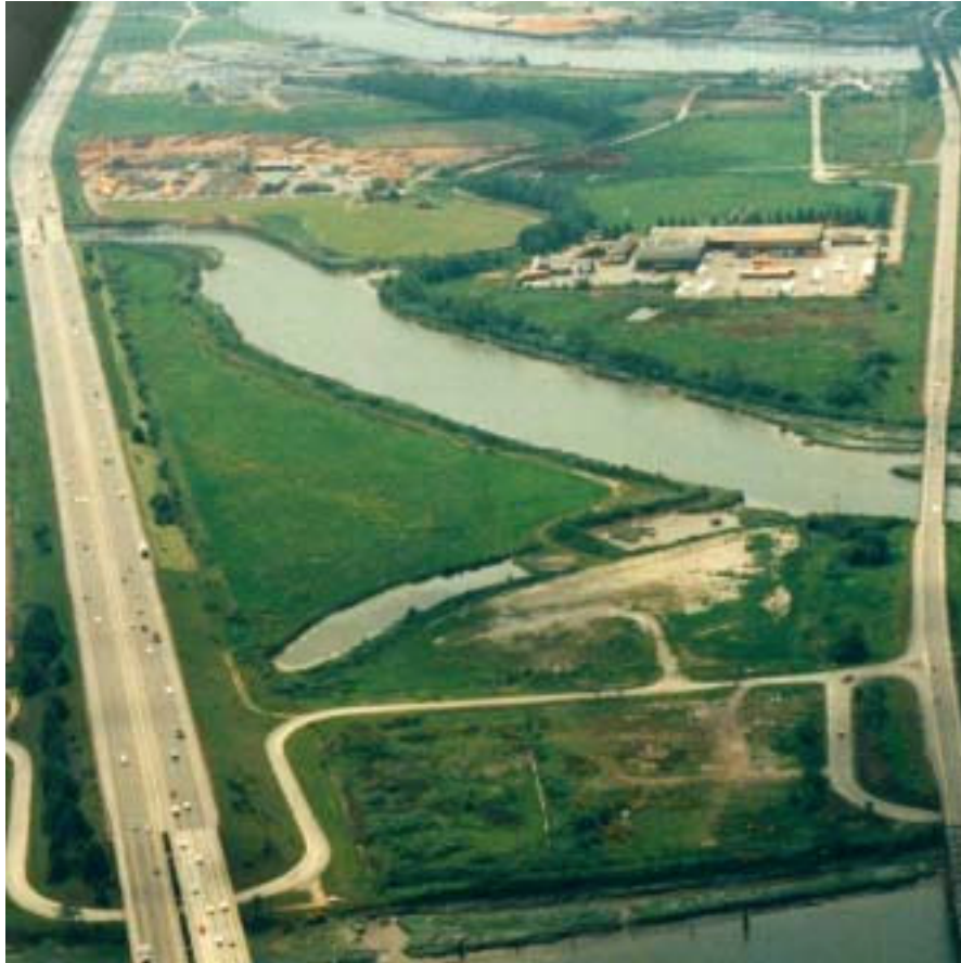
Figure 2 Union Slough Mitigation Project site, pre-construction; view to the south.
