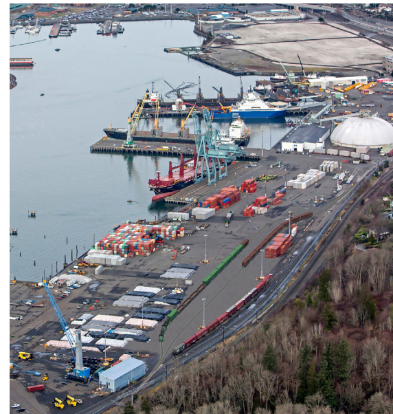
The Port's new double rail siding (depicted above) is anticipated for completion in November 2017.
